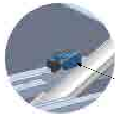
Fig.67 Limit switch in mcr PROLIGHT E type smoke vent
