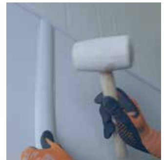
Step 4: Install Cover Profile
